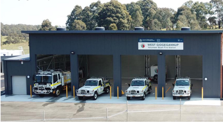
Gidgegannup Fire Station
